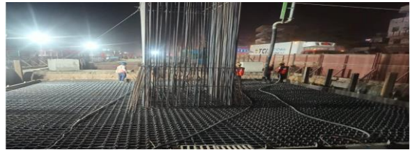
Fig. 5 Nighttime concreting and reinforcement work for a foundation, ensuring structural stability and load-bearing capacity
