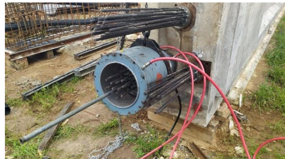
Fig. 9. Post-tensioning of multi-strand tendons using a hydraulic jack in a prestressed concrete element.
