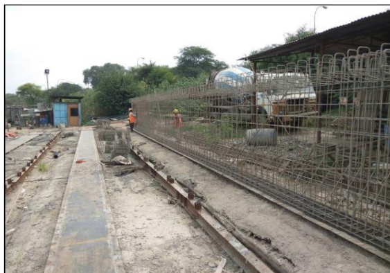
Fig. 11. Reinforcement cage assembly for a precast U-girder at a construction site,
