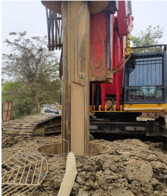
Fig. 1 Rotary drilling rig in operation for borehole excavation at a construction site, preparing the foundation for structural support
