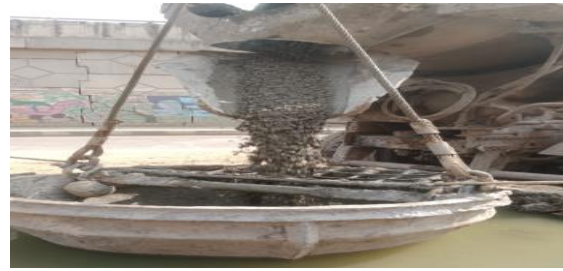
Fig. 3 Concrete being poured from a transit mixer into a suspended bucket for placement in deep foundation construction using the tremie method
