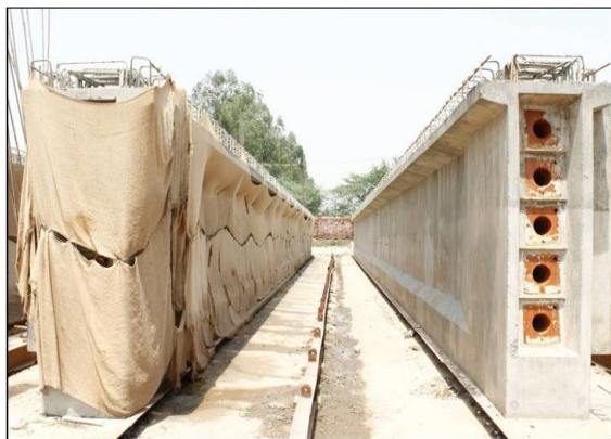
Fig. 10. Precast concrete U-girders stored at a construction site, with one covered for curing and the other showing post-tensioning ducts for cable installation
