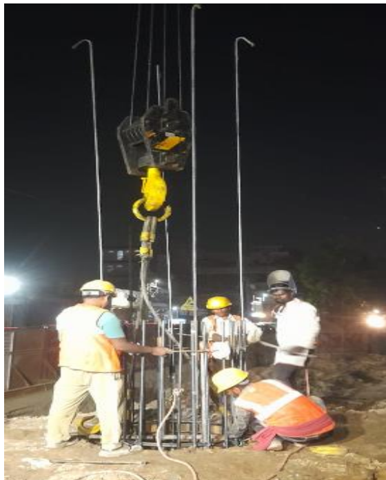
Fig. 2 Workers installing a reinforcement cage into a drilled borehole for deep
