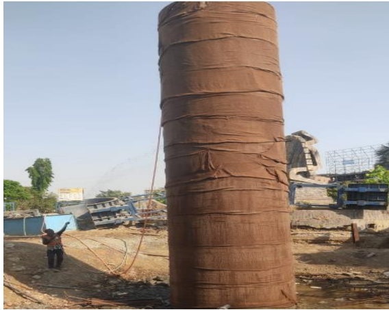
Fig. 6 Curing in progress: A concrete column wrapped in hessian cloth is kept moist to ensure structural strength and durability
