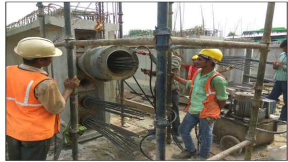
Fig. 12 . Workers performing post-tensioning of multi-strand tendons using a hydraulic jack in a construction site.
