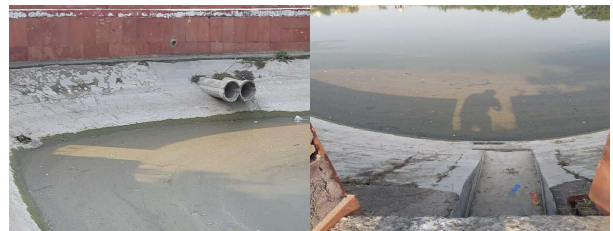
Fig.4 drains releasing water of some part of Sirsapur Delhi
